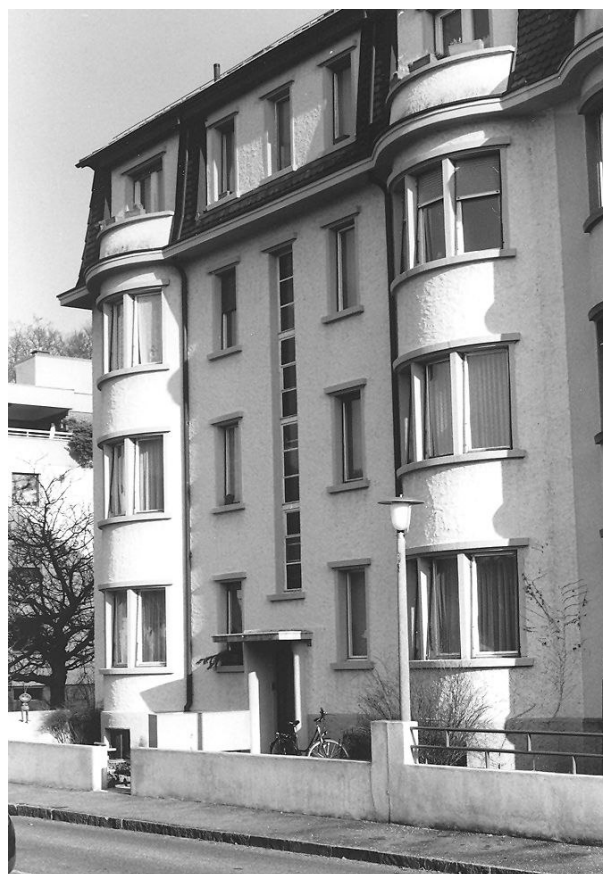
Details Treppenhaus, Erker
